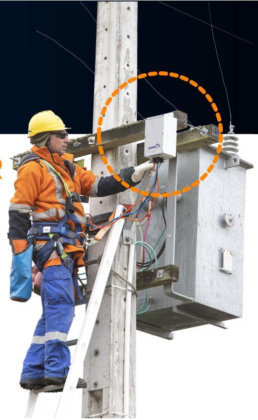
Pole Top Installation
