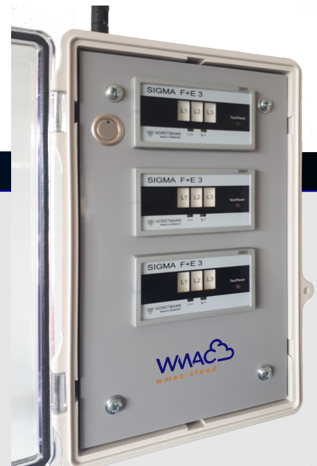
Sigma Fault Passage Indicator (FPI) with EdgeConnect
